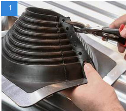
1 Select the appropriate Master Flash® Retrofit. If necessary, trim the opening to fit the pipe diameter.
