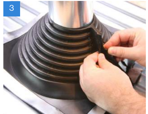
3 Secure Master Flash® Retrofit around the pipe using the plastic clamps provided to seal the flange.
