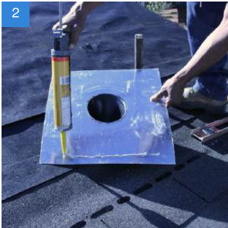
Apply sealant to the underside of the metal base.
