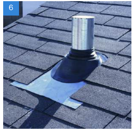
Finish installing the roof around the roof flashing.
