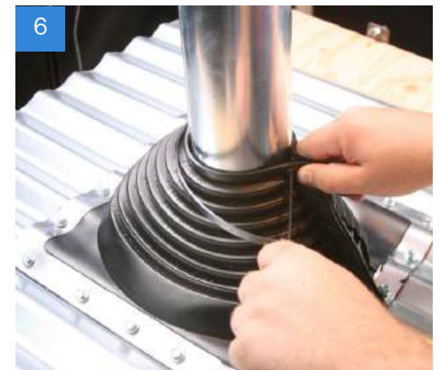
6 Drill holes in the flange for the fastening strap. Thread the strap through the hole. Tighten the fastening strap securely to ensure a proper seal. Additional sealant can be applied between the flange and the pipe.
