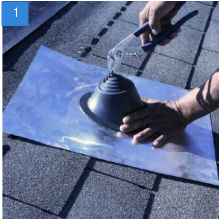
Adjust the flashing to the correct pipe diameter.
