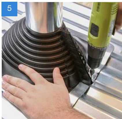
5 Use self-tapping screws to attach Master Flash® Retrofit to the substrate.
