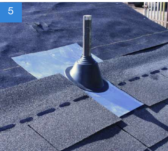
Install the roof tiles along the sides of the Master Flash®.
