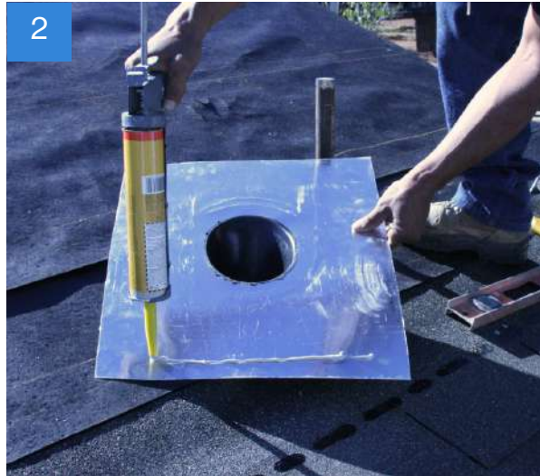
Apply sealant to the underside of the metal base.
