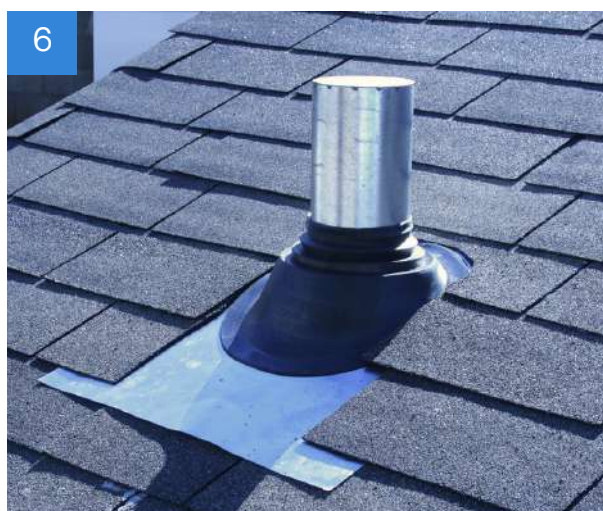
Finish installing the roof around the roof flashing.
