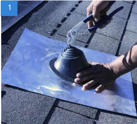
Adjust the flashing to the correct pipe diameter.
